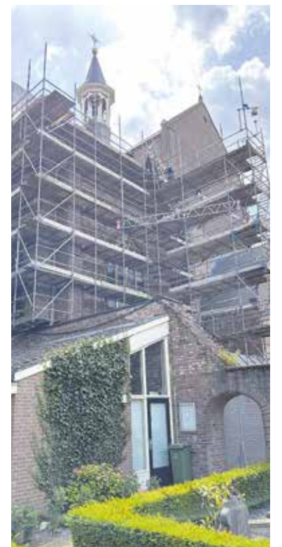
De restauratie is in volle gang.
